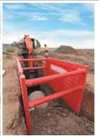
The 4M Series Trench Box can be handled by mid range excavators. These boxes are economical and ideal for general construction and utilities contractors. The 4M-60 is rated at 60kPa.
