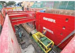
The 6M Trench Box is designed for large excavations and can be used in conjunction with Arch Spreaders. The 6M-40 is rated at 40kPa.
