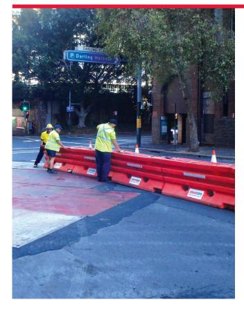
The Triton Barrier is an easy-to-use water-filled portable plastic barrier with an internal steel frame that provides work zone protection. The Triton Barrier has a convenient modular design that consists of a series of interlocking 2m barrier sections.
