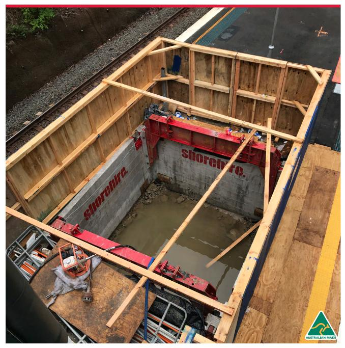
THE SHORE 5.2m-52 ALUMINIUM TRENCH BOX PROVES TO BE AN OPTIMAL CHOICE FOR THE INSTALLATION OF LENGTHY PIPE LENGTHS, BORING MACHINES, AND PUMP STATIONS, ESPECIALLY IN SCENARIOS NECESSITATING HEIGHTENED STRUT CLEARANCE. Its lightweight construction, coupled with 150mm thick panels, ensures unwavering durability in the face of rigorous demands.
