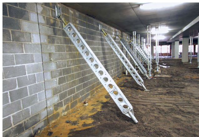
A - Angle of raking shore
