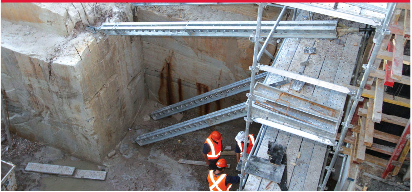
Shore Prop 100 Vertical Working Load Limit
