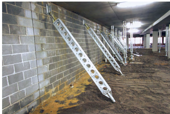
A - Angle of raking shore
