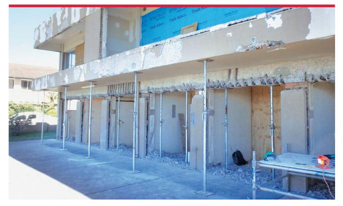
ACROW PROPS ARE HEIGHT-ADJUSTABLE, TEMPORARY STEEL SUPPORTS THAT ARE SUITABLE FOR VARIOUS PROPPING TECHNIQUES IN A WIDE RANGE OF CONSTRUCTION SETTINGS. THEY ARE DESIGNED AND MANUFACTURED TO FULLY SATISFY THE REQUIREMENTS OF THE AUSTRALIAN FORMWORK CODE.
