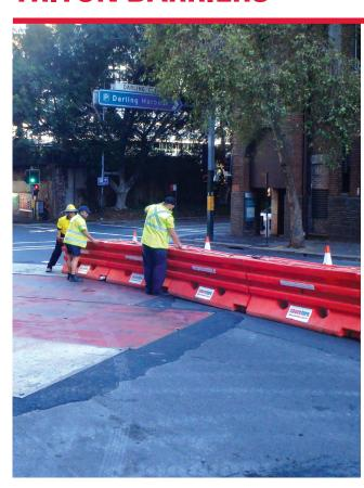
The Triton Barrier is an easy-to-use water-filled portable plastic barrier with an internal steel frame that provides work zone protection. The Triton Barrier has a convenient modular design that consists of a series of interlocking 2m barrier sections.
