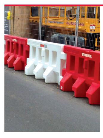
Whether you are looking for a traffic delineator for a slow-speed work zone or pedestrian control, our SH 2000 Water Filled Barrier will meet your needs.
