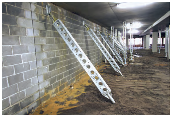
A - Angle of raking shore
