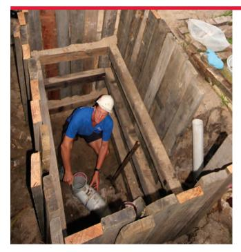
Shore Hire carry a large range of Timber Shoring, including Runners, Walers and Trench Jacks. Timber Shoring is a trench support system for pipe laying maintenance and excavations that can be installed by hand, without the use of excavators. It is a very adaptable system suitable for many different situations including small access areas and the presence of cross services within the excavation.
