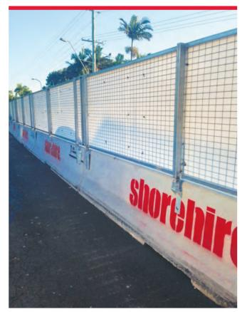
Concrete T-Lok barriers are designed for traffic diversion and separation. The T-Lok precast Concrete Barrier has an Austroads Safety Barrier Acceptance Panel (ASBAP) approval to 80km/h as a temporary redirective longitudinal barrier.
