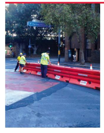
The Triton Barrier is an easy to use water filled portable plastic barrier with an internal steel frame for work zones. The Triton Barrier has a convenient modular design that consists of a series of interlocking 2m barrier sections. Triton Barrier provides approved work zone protection.
