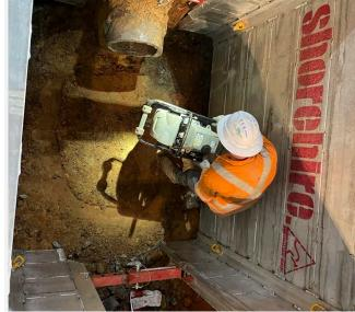
SHORE HIRE'S MANHOLE ALUMNIUM SHORING BOXES ARE AN INCREDIBLY VERSATILE AND SAFE TRENCH SHORING SYSTEM FOR GENERAL CONSTRUCTION AND UTILITIES CONTRACTORS.
