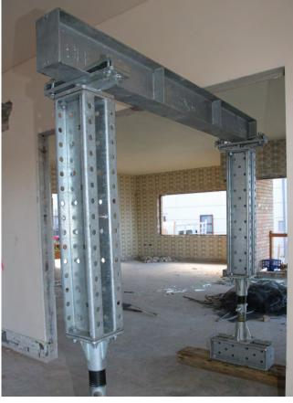
Needle Beams are used in propping and needling applications, and our engineers often specify their use to spread loads whilst supporting slabs. Our needle beams have been reinforced with additional stiffener plates and galvanised for protection.
