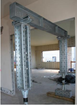
Needle Beams are used in propping and needling applications. Engineers often specify their use to spread loads whilst supporting slabs. All of our needle beams have been reinforced with additional stiffener plates and galvanised for protection. Available in various sizes in both universal columns and universal beams.
