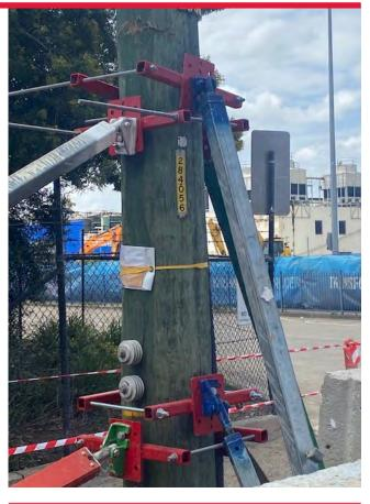
Shore Hire's Power Pole Bracket is a custom-built solution designed to be used in pole propping applications.
