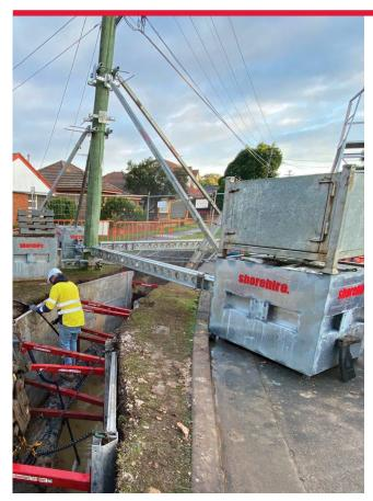
SHORE HIRE'S POWER POLE CLAMPS ARE SUITED FOR POLE PROPPING APPLICATIONS. THE BRACKETS THEMSELVES ARE SUITED FOR POLES WITH A DIAMETER BETWEEN 250-530mm BUT A CUSTOM SOLUTION CAN BE CREATED IF NECESSARY.
