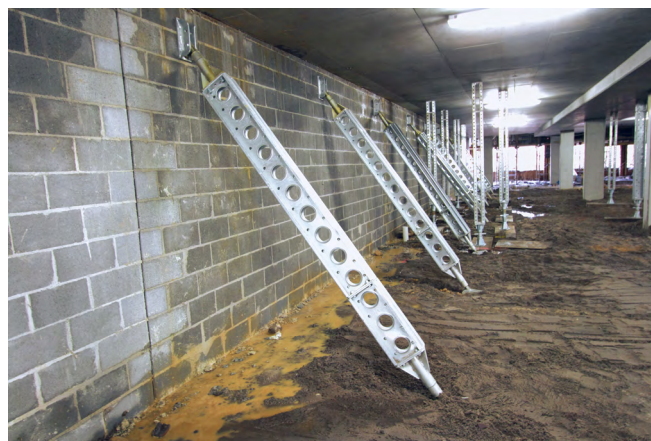
A - Angle of raking shore
